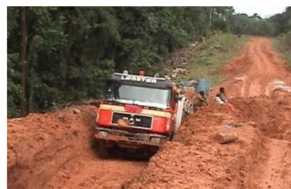
POOR ROADS ARE HINDERING AGRICULTURAL DEVELOPMENT (PHOTO: MISSION LIBERIA)
