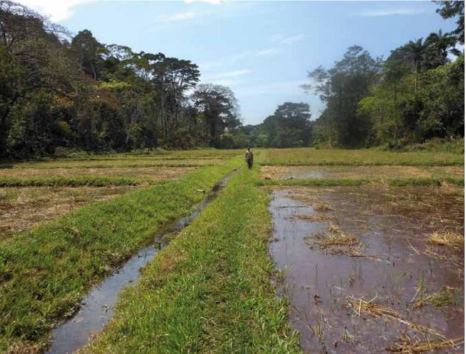
Fig. 30 Planting of cover plants to protect the structure from erosion damages
