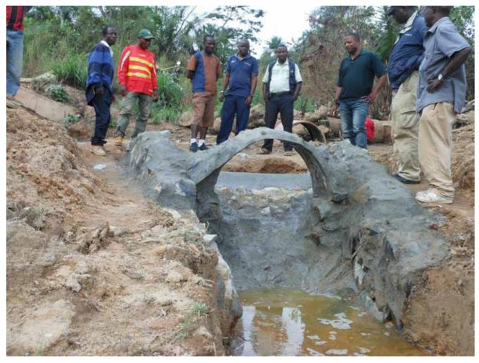
Fig. 23c Completed work needs at least three days curing (splash water over it every hour).
