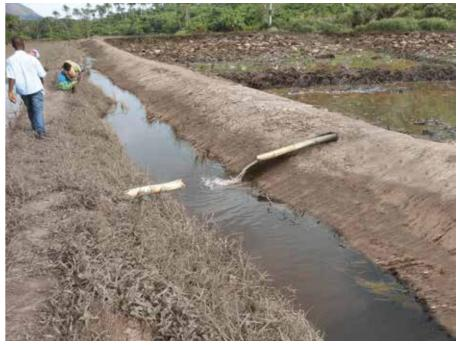
Fig. 28 Bamboo or PVC Pipe per plot for drainage
