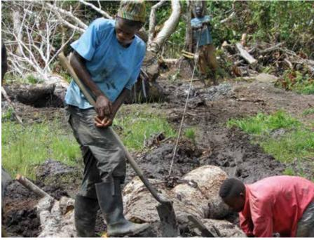
Fig. 18 De-stumping Abura tree with the help of cable pulling device "Come Along"
