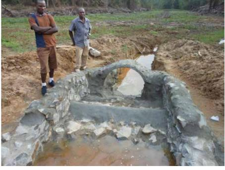
Fig. 23b Fill joints between rocks with quality mortar. Add a second layer if your stones/rocks are lying flat. Use any formwork to construct arch bridge.
