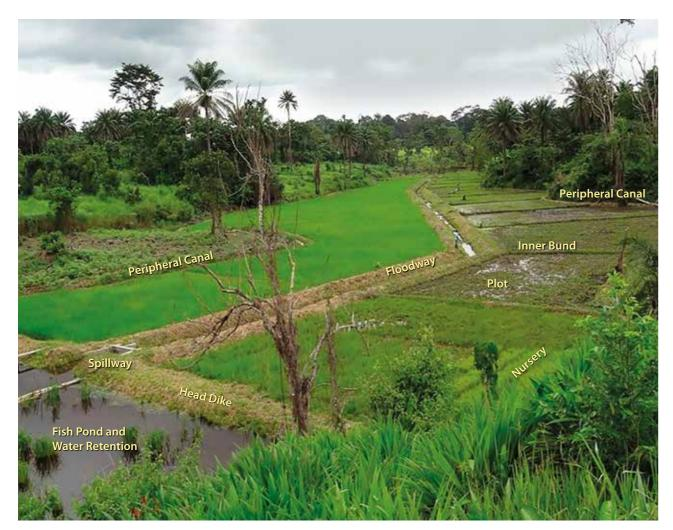
Cover photo: The Main Components of Irrigation Schemes
