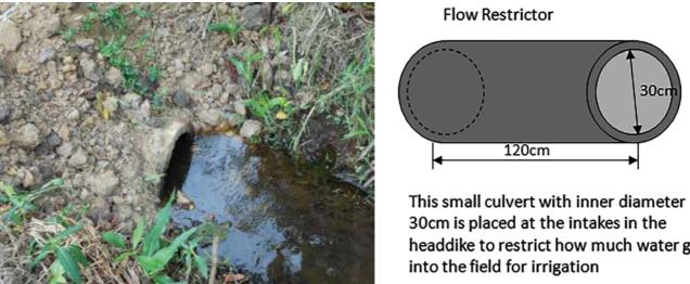
Fig. 24 Flow Restrictors at Intakes of Supply Canal
