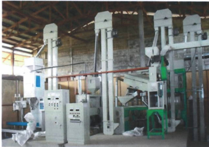
Photo 22: Rice mill factory
