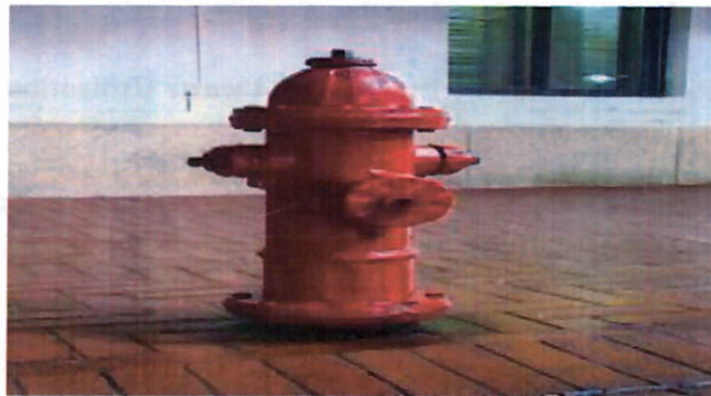
Fig 48 A typical fire hydrant
